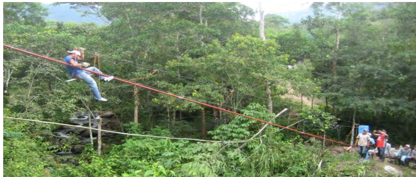
An ETAP student learning to put up a suspension pipe bridge with a sky hook.
